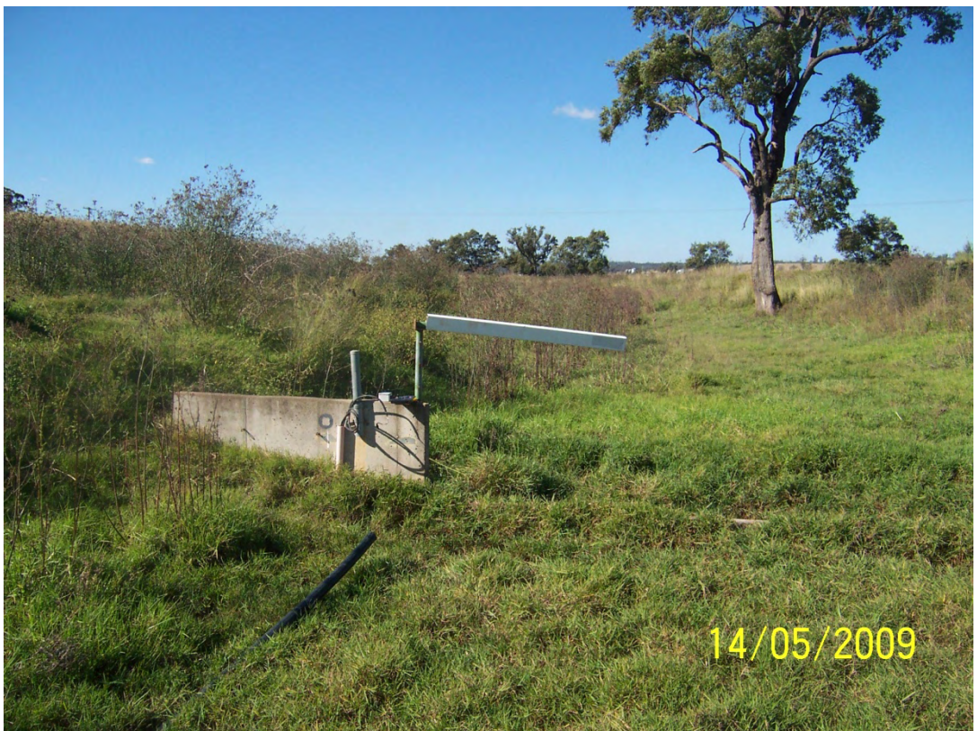
Plate 2: Abandoned Monitoring Weir Chainage 60
